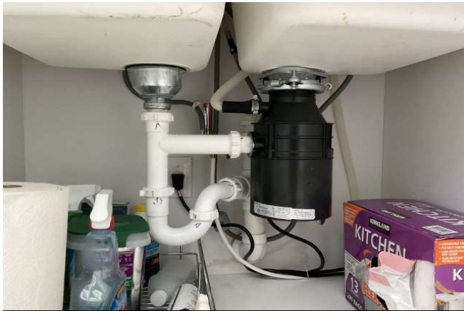
Plumbing - Kitchen Sink
