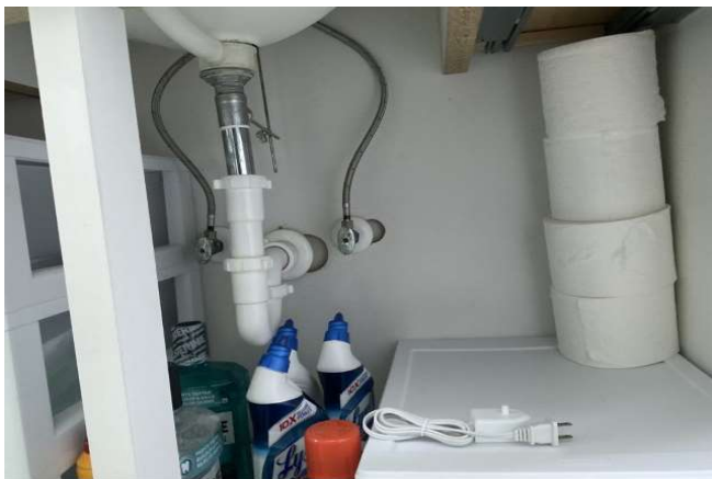
Plumbing - Master bath right sink
