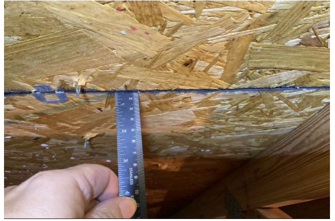
Roof Deck Thickness - 7/16ths
