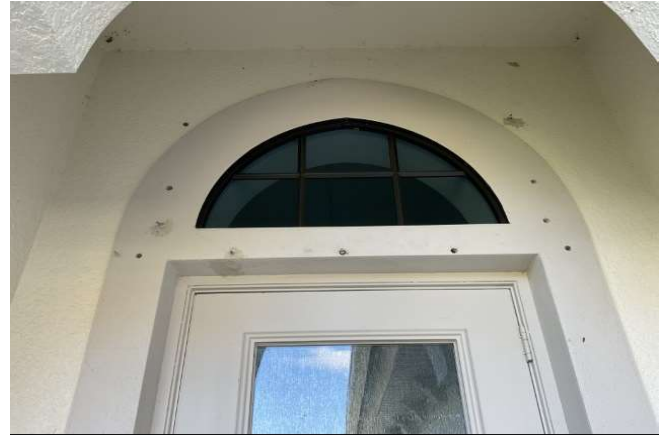
Front Door Storm Shutter Attachments
