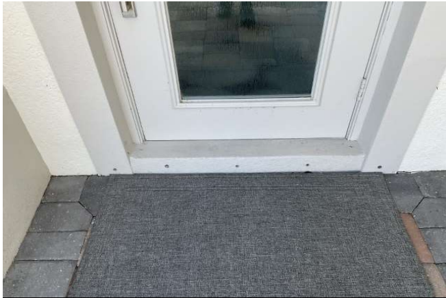
Front Door Storm Shutter Attachments
