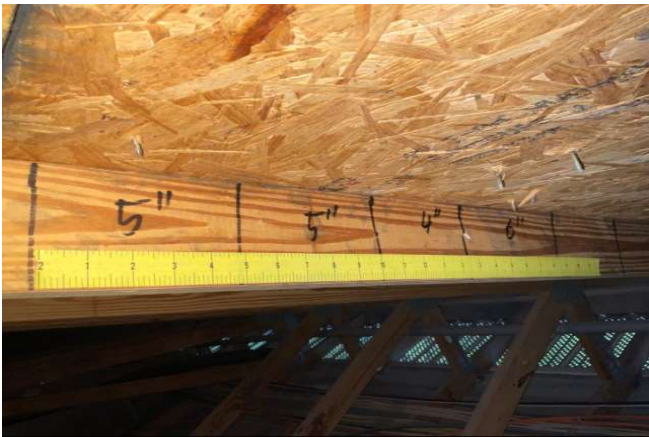
Roof Deck Connection - Nail Spacing
