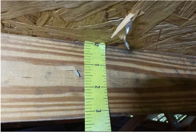
Roof Deck Connection - 8D Nail
