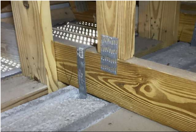
Roof to Wall Connection - Single Wraps - Front
