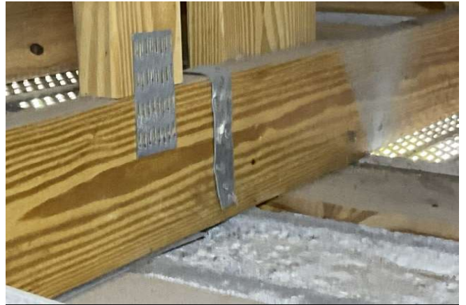
Roof to Wall Connection - Single Wraps - Back
